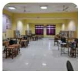
Power System Lab
